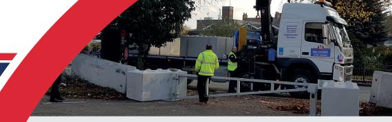
Blocks can be lifted and installed into place quickly using standard construction lifting equipment such as small cranes and forklifts. The interlocking mechanism of the blocks means each one fits together smoothly – and won't become displaced accidentally.
